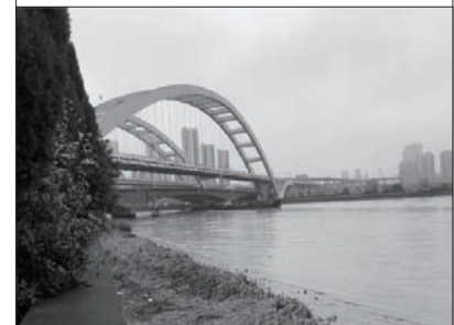
deformation monitoring of bridges and tunnels
