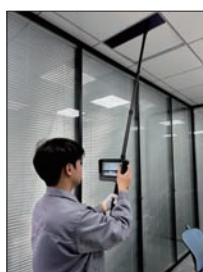
ceiling duct inspection
